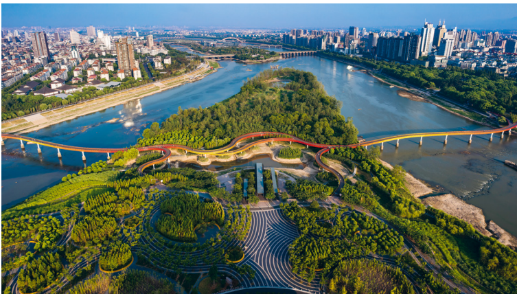
Figures 4-1 to 4-3 The three images (from top to bottom) show Yanweizhou Park during a 100-year flood event, a 20-year flood event, and during the dry season. © Turenscape Academy
