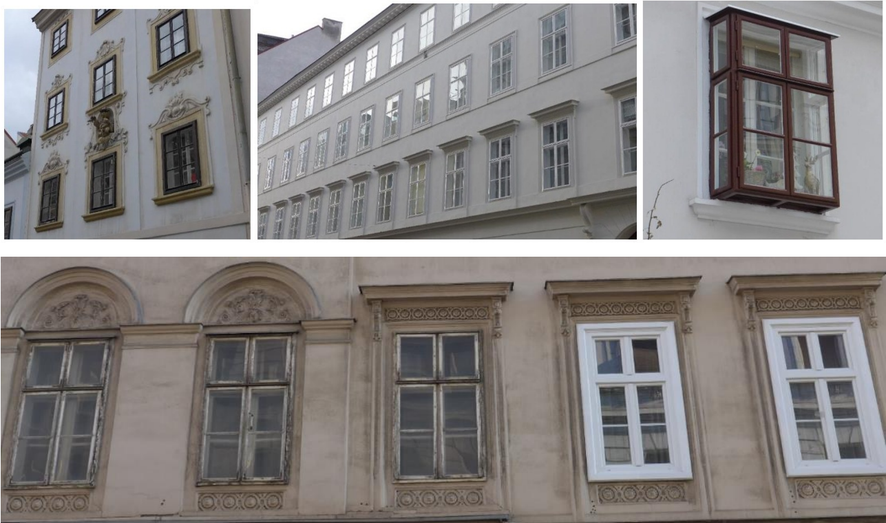
Fig 3. Beautiful casement windows (upper row) versus inconsistent appearance of a façade with casement windows of little maintenance and incongruous replacements by multi-layer insulation-glass windows made of plastic (© P. Schober).
