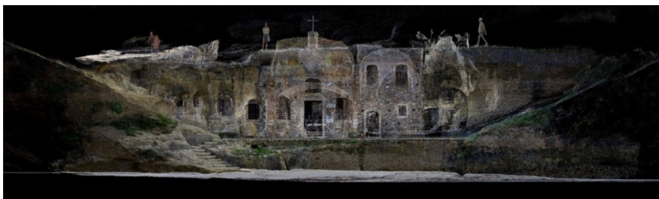
Fig. 1. Main elevation. Point cloud post-processing. (© L. Pizzonia).
