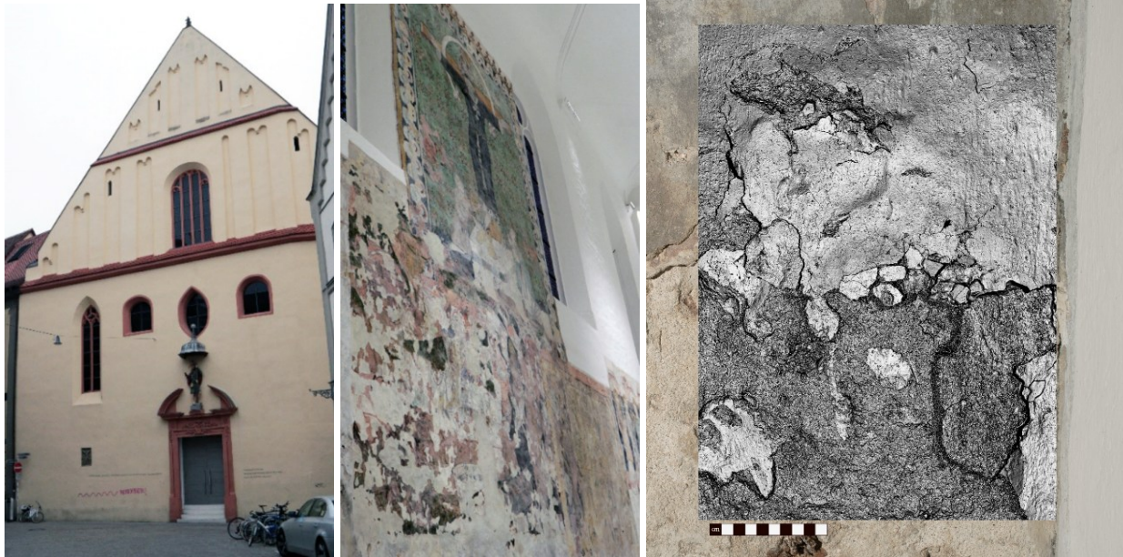
Fig. 3. Left: A street view of the former Dominican church of St. Christopher in Bamberg. Centre: Wall painting inside the former Dominican church showing a Volto Santo. Right: Reference area of the medieval wall painting taken by the structured light scanner laid on top of an orthogonal colour photography (© Leander Pallas).
