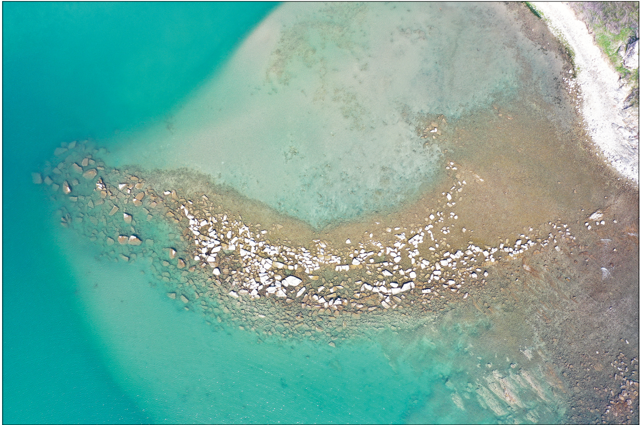
Fig. 13 Abdera. South enceinte. Harbour structure no. 4. Southwestern breakwater after sea level receding. – (Photo K. Darakis, 10.03.2021).
