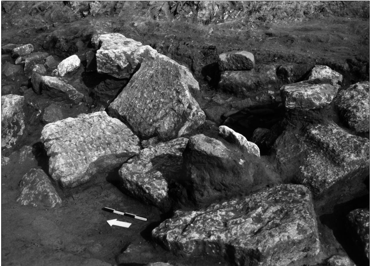
Fig. 11 Abdera. South enceinte. Harbour structure no. 3 (quay). Breakwater blocks west of the quay. – (Photo C. Kallintzi, 1993).
