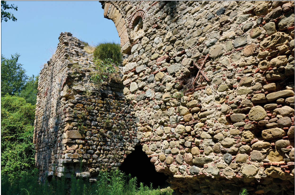
Fig. 4 Anastasioupolis. Harbour gate from the northeast. Late Byzantine construction according to tile monograms erected over older, probably early Byzantine, masonry. – (Photo Th. Schmidts).
