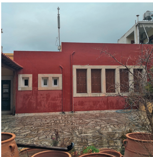
Fig. 32 The Archanote Center for the Elderly ("KAPI"), a modern construction painted in "Minoan red". (Photo by the author)
