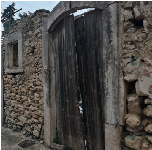
Fig. 22 Arched stone frames and other monumental elements in local houses. (Photo by the author)
