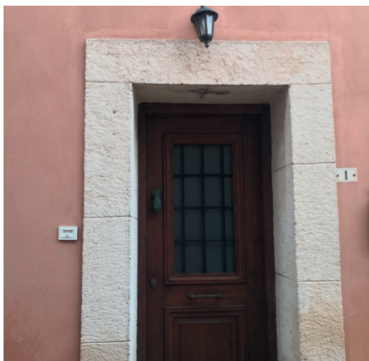
Fig. 29 Door frame in stone. (Photo by the author)
