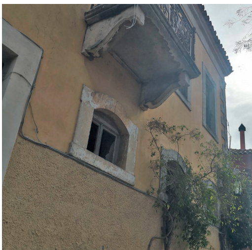
Fig. 30 Architectural elements in stone. (Photo by the author)
