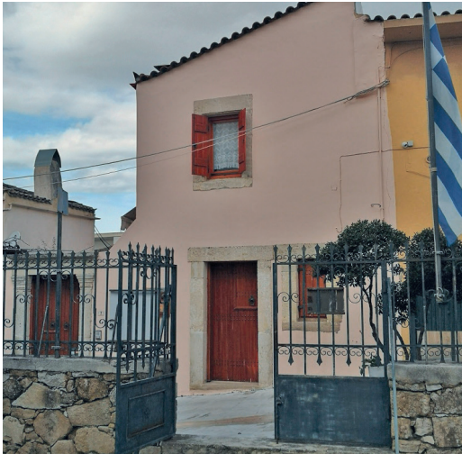
Fig. 45 Uncovered pelekia (stone frames) in a restored house opposite the Archaeological Museum of Archanes highlight the importance of the local conservation program. (Photo by the author)
