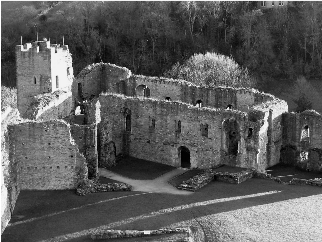
Abb. 9 Scolland's Hall, Richmond castle, viewed from the north. To the right is the main entrance to the hall at first floor level, while the lower hall is entered through the arch to the left at ground floor level (Matthew J. Strickland).
