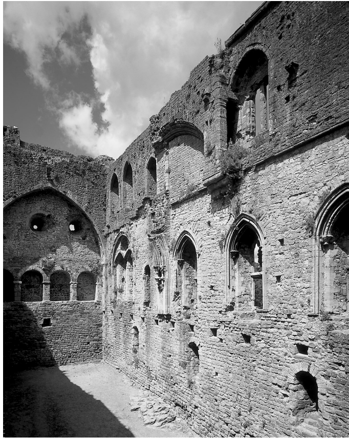
Abb. 4 Interior of the great tower at Chepstow, looking west through the doorway in the east wall, and showing the two oculi and arcade of niches decorating the first floor (Cadw, Welsh Assembly Government, Crown Copyright).
