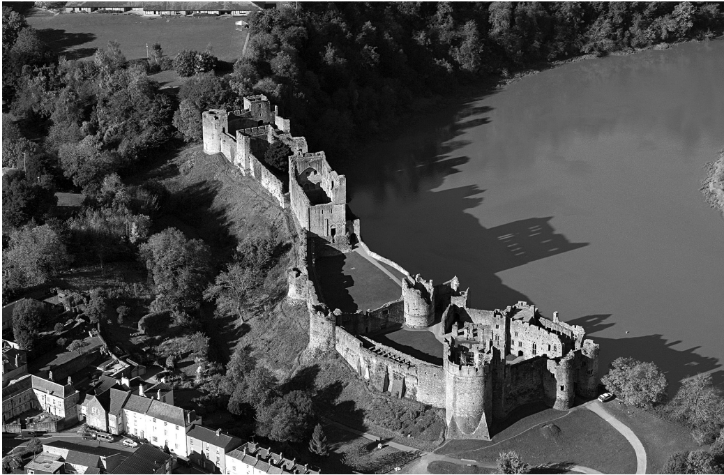
Abb. 1 Chepstow castle, Gwent, from the east, with the eleventh-century great tower in the centre. The niches and two oculi on the west wall are visible below the supporting arch added during Earl Roger Bigod's remodelling of the great tower between 1293 and 1300. In the lower bailey is the earl's new domestic range (to the lower right) (CADW, Welsh assembly Government, Crown copyright).
