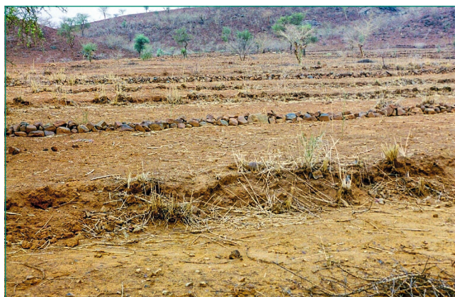
Figure 18 – Piled up stones form small dams to retain the rainwater – the picture was shot nearby Sabouna (Yatenga)
