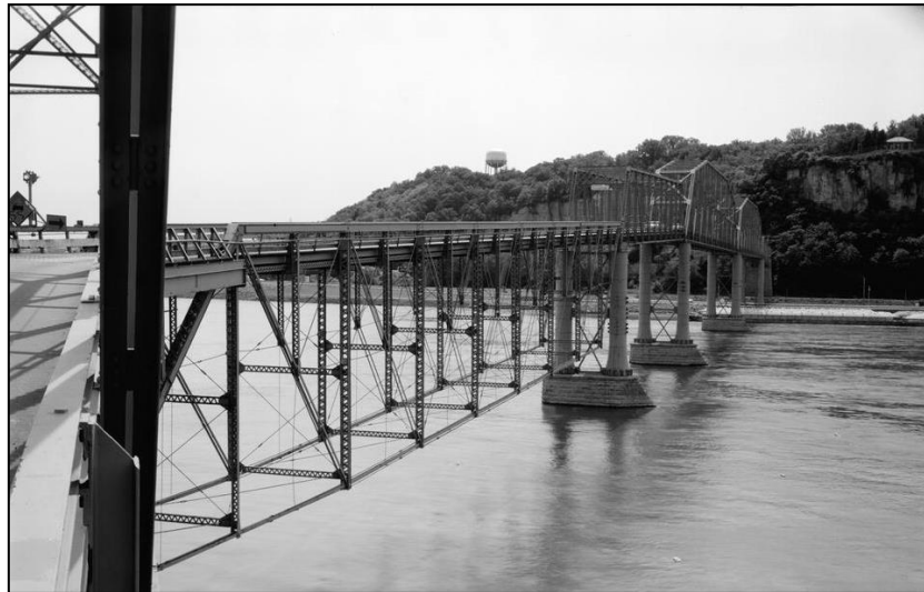
Fig. 1. Eagle Point Bridge, Dubuque IA, 1902 (HAER IA-2-56). (Image Source: https://www.loc.gov/re-source/hhh.ia0114.photos/?sp=56&q=Eagle+Point+Bridge )
