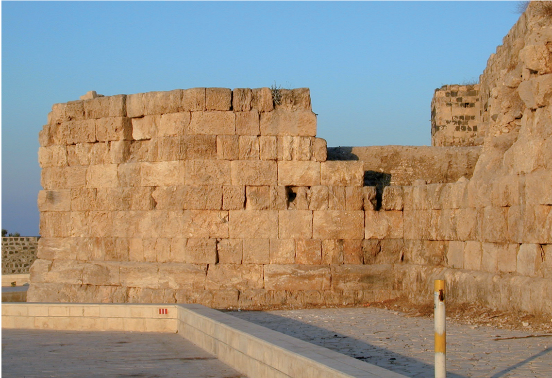
Fig. 2: Tower 3 with bricked up sally port.
