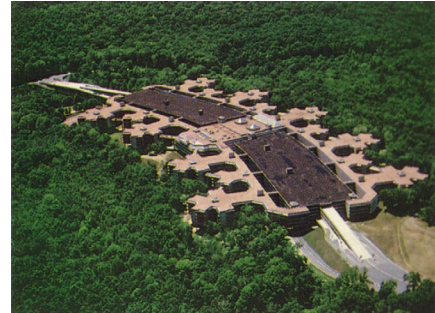
10| Union Carbide Headquarters, Danbury (CT), 1982, Kevin Roche, John Dinkeloo and Associates
