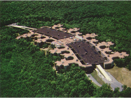
10| Kevin Roche, John Dinkeloo and Associates, Union Carbide Headquarters, Danbury, Connecticut, 1982
