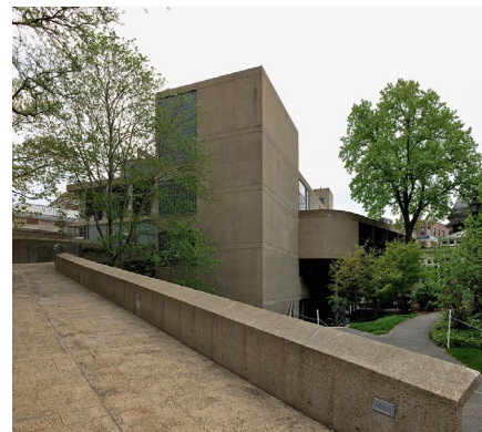
33| The Carpenter Center for the Visual Arts at Harvard University, Cambridge (MA), 1962, Le Corbusier
