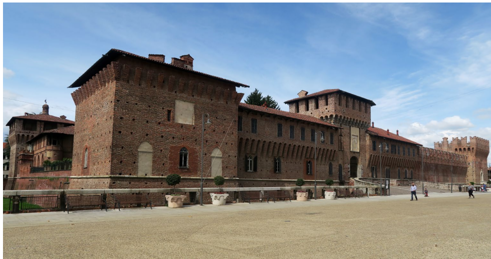
Fig. 6. Castello Visconteo-Sforzesco, Galliate (Novara)
