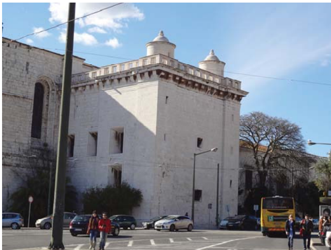
Fig. 12 Exterior view of the capela mor . Photo: A. Jordan Gschwend.
