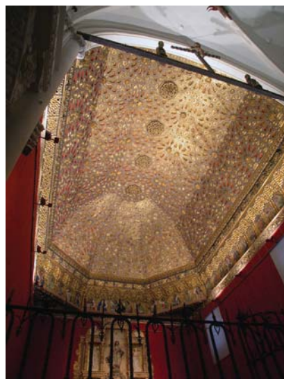
Fig. 2 Moorish ceiling of the present church, Monastery of Santa Clara, Tordesillas, 14 th century.
