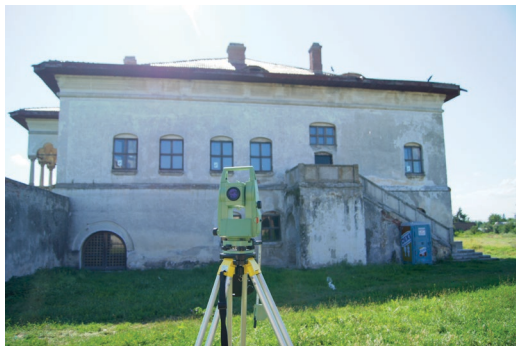
Fig. 20 Total station set up.
