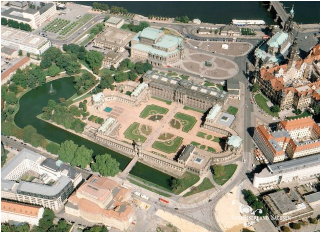
Fig. 5 Aerial view of the Dresden Zwinger: at the right the court church and the residential castle with the adjoining Taschenberg Palace is situated; above, between the Zwinger courtyard and the river Elbe, the 2nd court theatre, today known as 'Semper-Oper' (photograph: first decade of 21st century).
