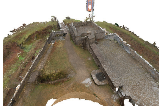
Fig. 35 Ginsburg, 3D model, view on the courtyard and the basement of the 'Palas' (2012).
