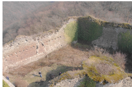
Fig. 29 View over castle Rauschenburg showing remains of the turret and the walls (2012).
