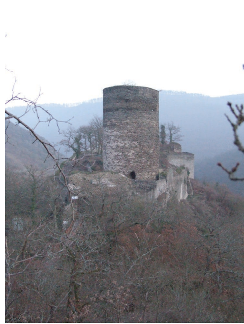
Fig. 18 The round tower of Castle Stahlberg from the northwest (2005).
