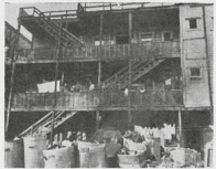
EAST SIDE, just east of the railroad tracks. Though the percentage of multiple dwellings is small, too many of the tenements are of flimsy wood. Garbage is collected only twice weekly.
