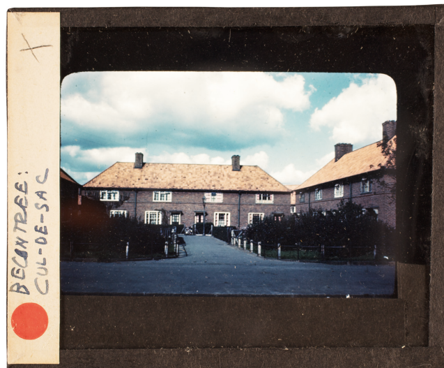
79] Unidentified photographer, "Becontree: Cul-de-sac," undated, lantern slide, 3.25 in. × 4 in. (8.26 cm × 10.16 cm), in box "9 of 21," William and Catherine Bauer Wurster Papers, Environmental Design Archives, University of California, Berkeley.
