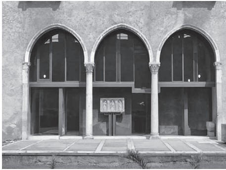
Abbildung 150. Carlo Scarpa, Museo Castelvecchio, Verona, 1954–64, Fassade (Detail)
