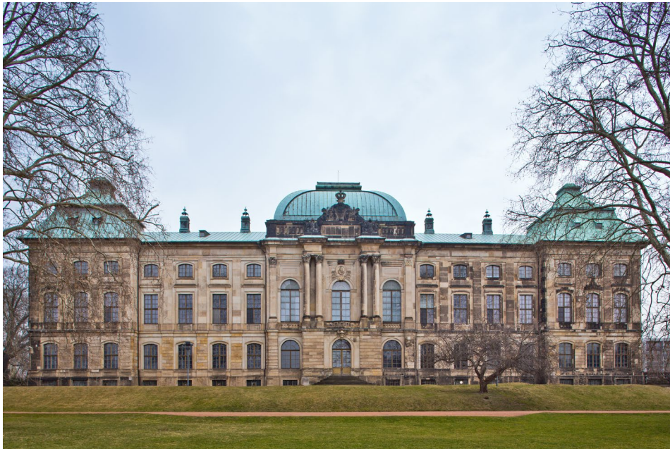
Fig. 2. The Japanese Palace in Dresden, south front facing the Elbe River.
