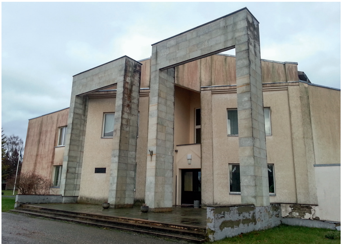
Fig. 3: Administrative-cultural centre of the Lümända State Farm, architect Veljo Kaasik, completed in 1986 (2016).
