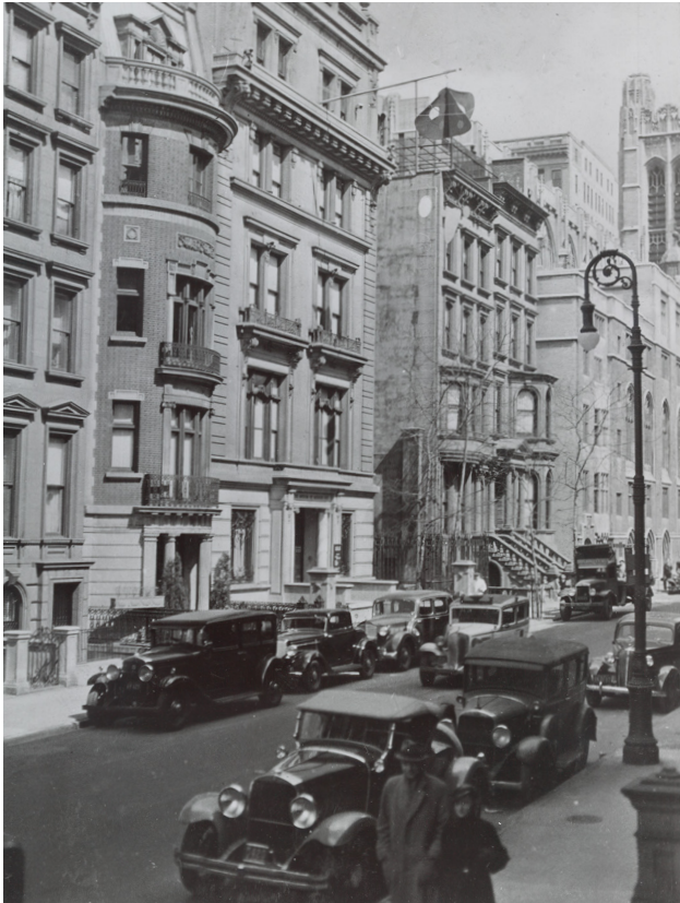
17 Beaumont Newhall, facade of the original townhouse of the Museum of Modern Art at 11 West Fifty-Third Street, showing a Calder mobile displayed in the exhibition “Cubism and Abstract Art,” 1936. New York, The Museum of Modern Art Archives.
