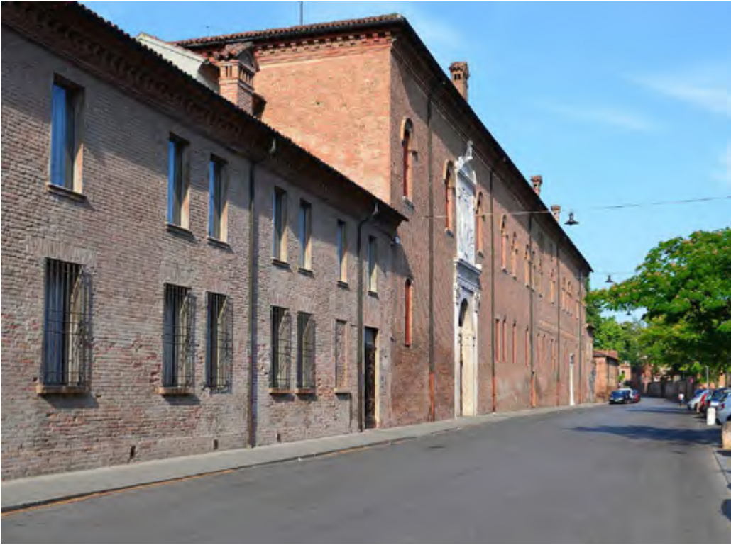
11. Palazzo Schifanoia, Ferrara, general view.
