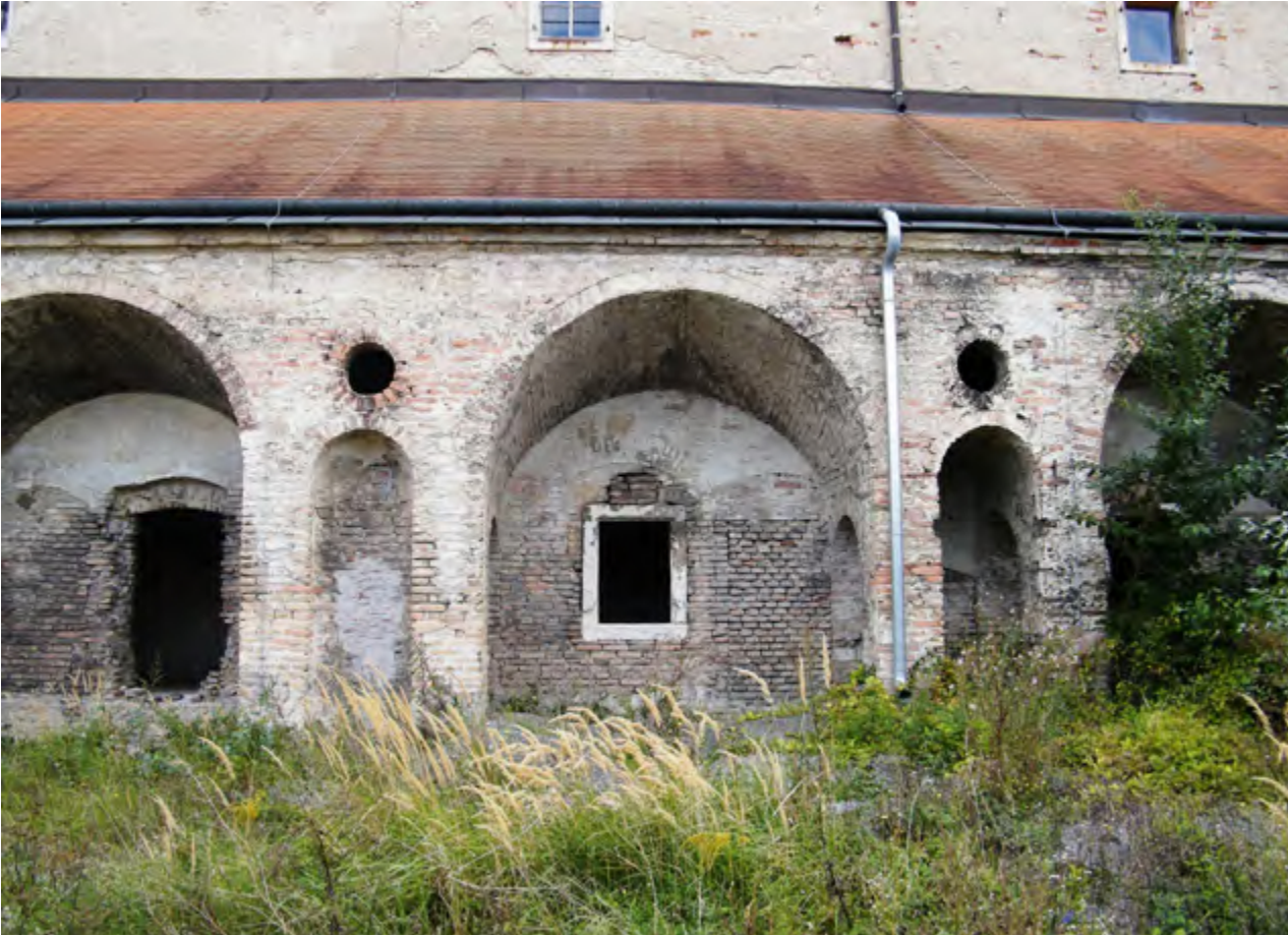
3. The fishponds in the lateral courtyard of the Neugebäude.
