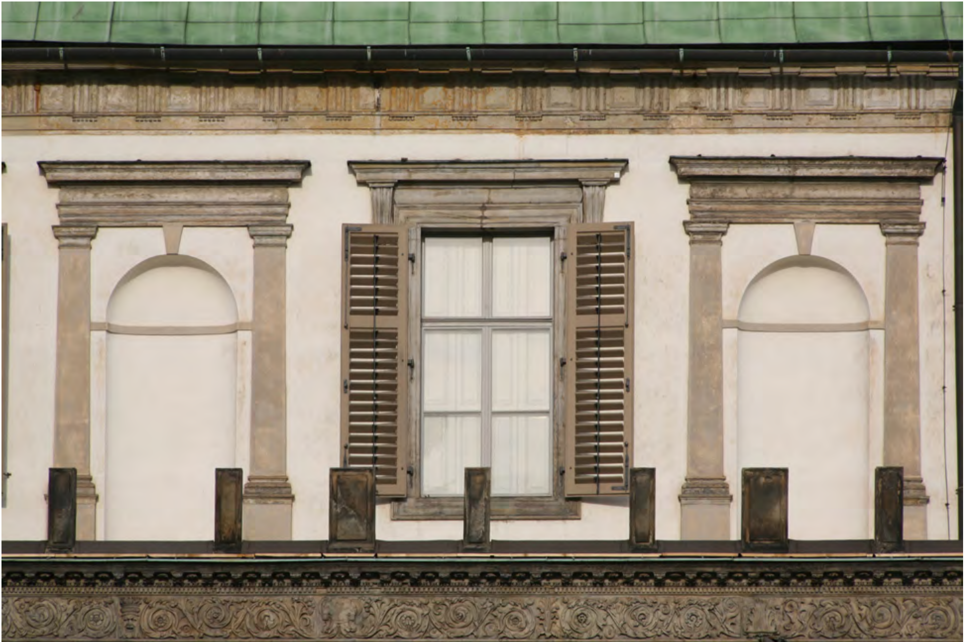
4. Photograph of the upper facade of the Belvedere, showing niche and window.
