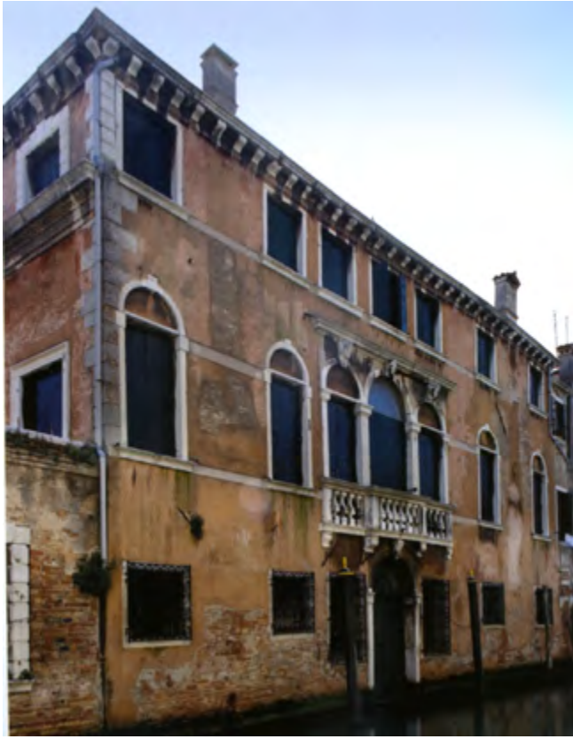
9. Antonio Gaspari, Casino Zane, facade on Rio Marin, 1694–98.
