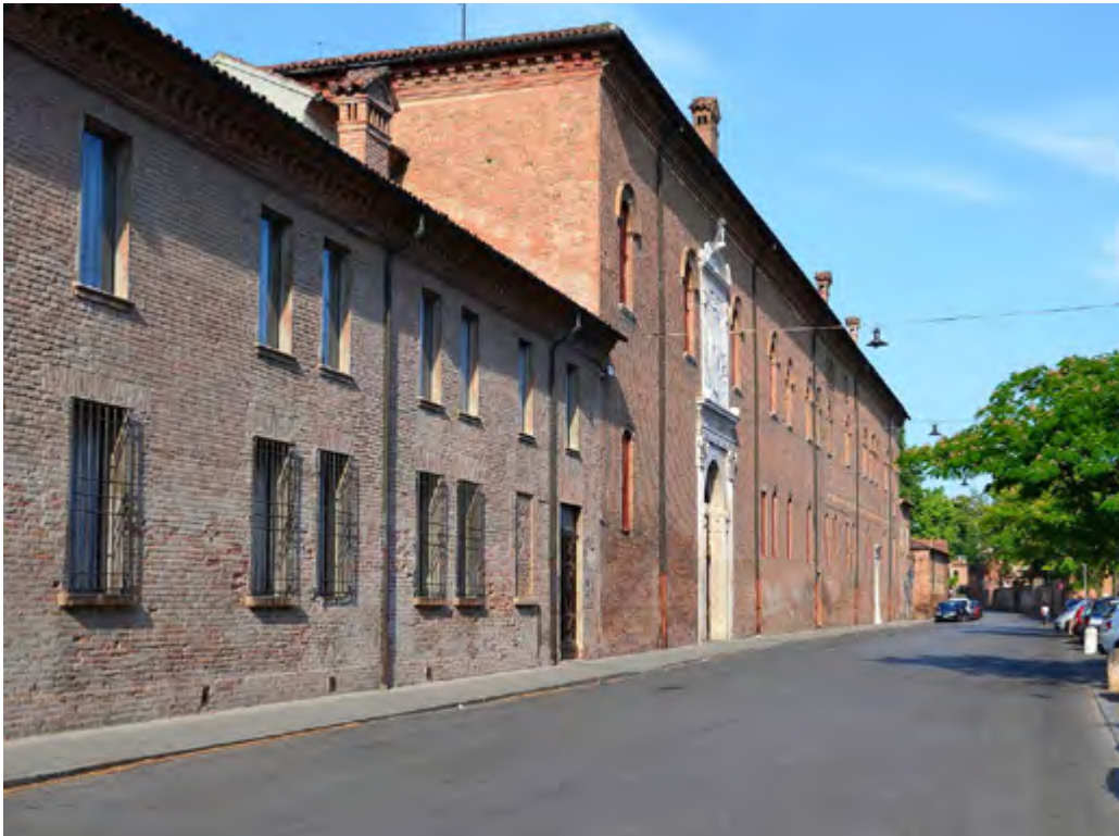
11. Palazzo Schifanoia, Ferrara, general view.
