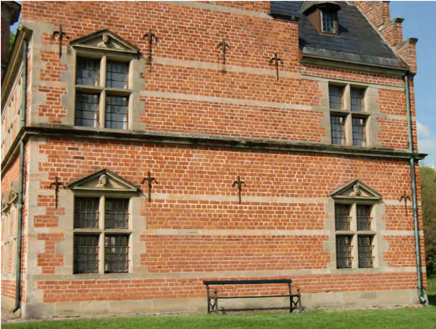
1. Frederik II's Bath House from 1580 near Frederiksborg Palace. The red brick walls with white bands of sandstone and the triangular frontons with human heads are typical of Danish Renaissance architecture, inspired by the Netherlands.
