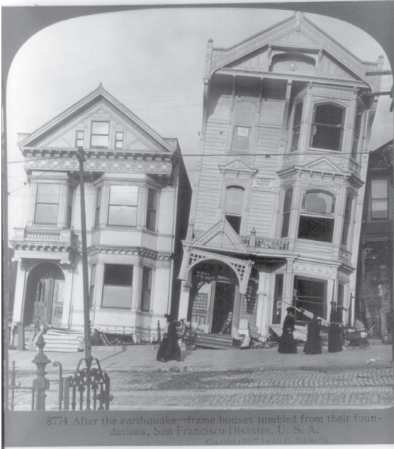
156. H. C. White, After the earthquake – frame houses tumbled from their foundations, San Francisco Disaster, U.S.A., 1907. Hälfte einer Stereographie.
