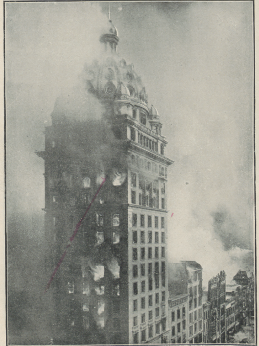
BURNING OF THE CALL BUILDING APRIL 18TH Haley, photo This tower-like structure, which is 315 feet from sidewalk to tip of dome, suffered small damage from the earthquake. Its frame was unhurt by fire and the interior is being speedily restored.
