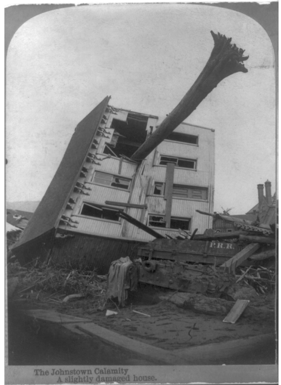
155. George Barker, The Johnstown calamity. A slightly damaged house , 1889. Hälfte einer Stereographie.
