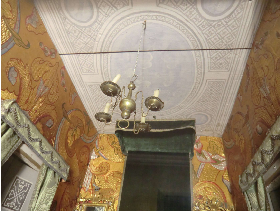
Fig. 11 Offene Tafel . Gilded-leather wall cover (original size), geometrically ornamented ceiling in imitation of stucco, chandelier and draperies above the doors.
