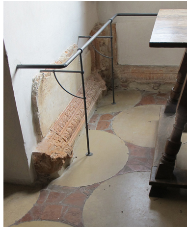
Fig. 7 Schloss Neuburg am Inn, White Marble Chamber, northern bay of the eastern side, remains of terracotta moulding in situ .
