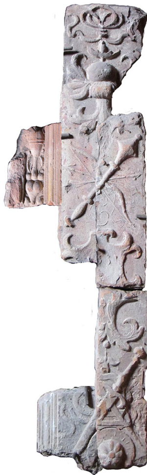
Fig. 5 Schloss Neuburg am Inn, fragments of a pilaster strip, probably from a door jamb, dated '1531', photomontage.
