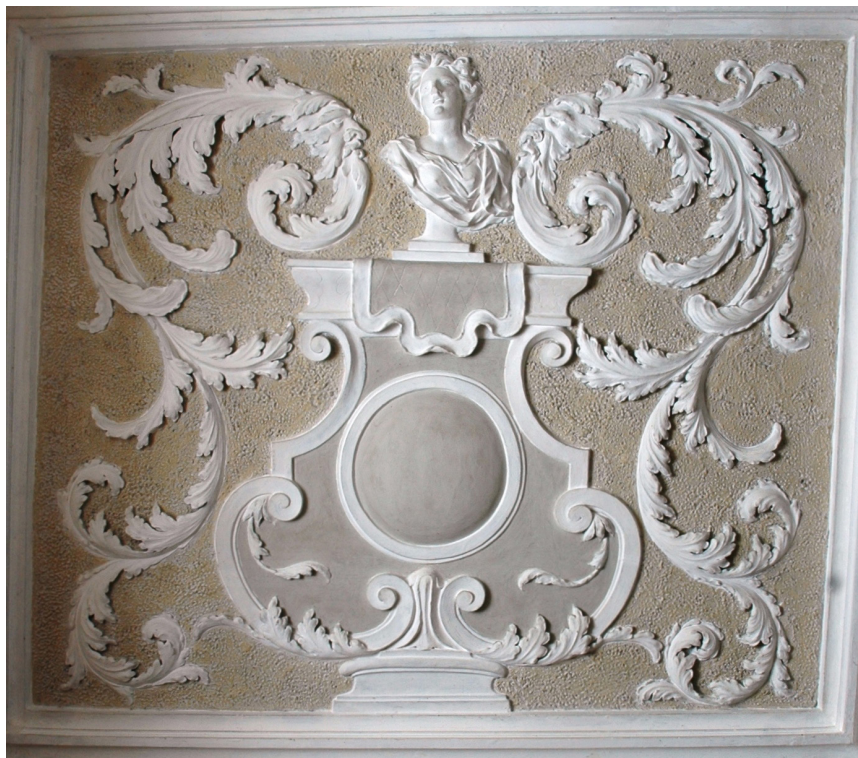
Fig. 7 Ludwigsburg palace, stucco ceiling in the ground floor vestibule, 1710.
