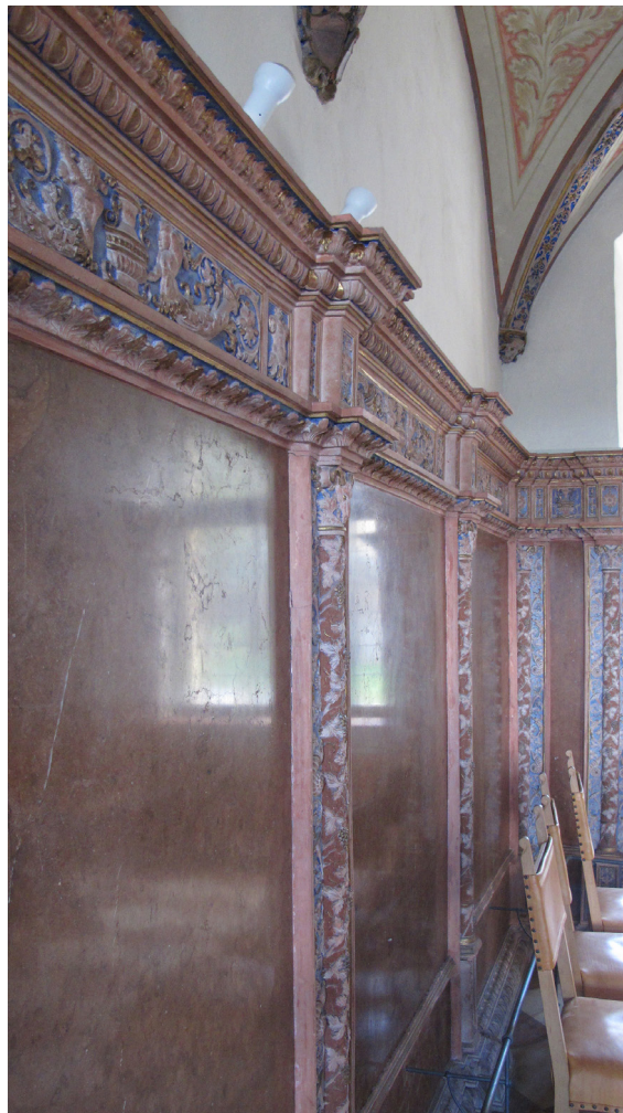
Fig. 14 Schloss Neuburg am Inn, Red Marble Chamber, wall panelling reconstructed, present state.
