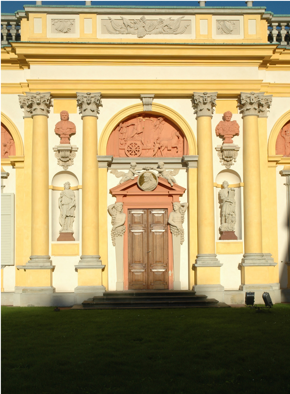
Fig. 2 Wilanów, façade of the King's Gallery.
