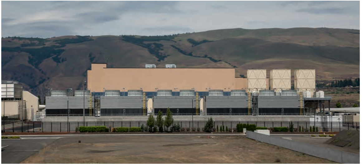
Abb. 4: Google Data Center – The Dalles, Oregon | Fig. 4: Google Data Center – The Dalles, Oregon (2015)
