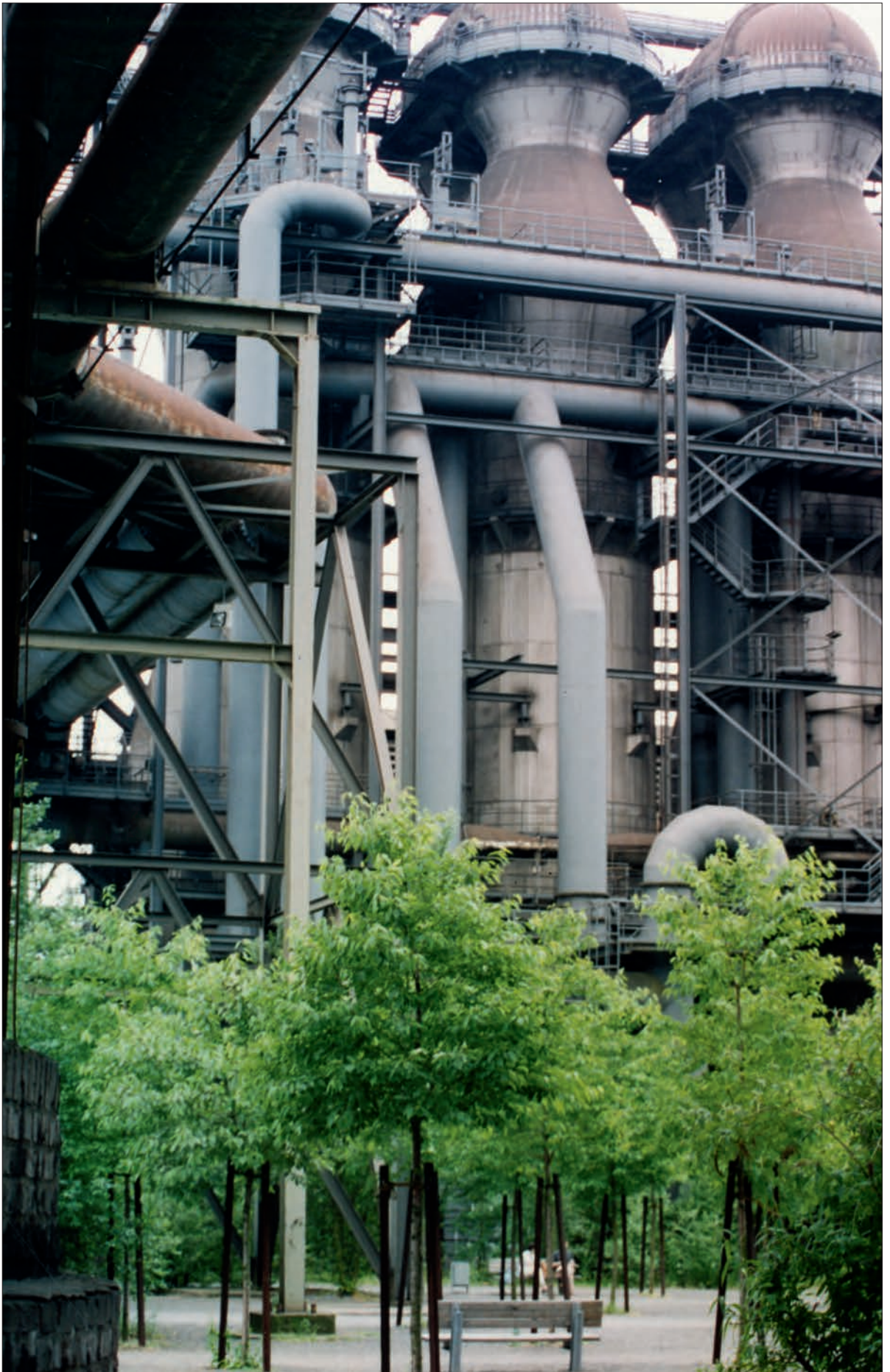
Fig. 3: Duisburg Nord entry plaza (Photo by the author)
