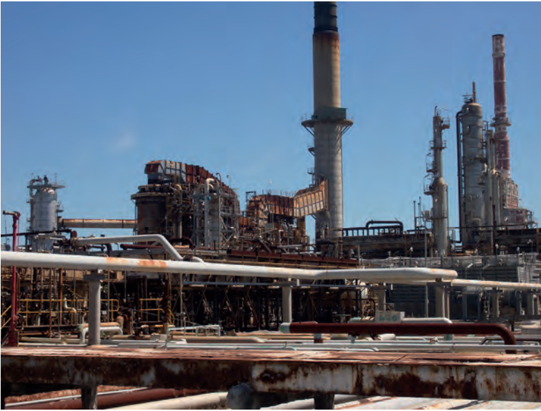
Fig. 1: View of fuel processing infrastructure buildings, Caltex Oil Refinery Botany Bay Sydney (2016)
