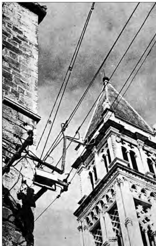
Fig. 3: Nada Orel, Electrical installations in the centre of Trogir, 1976, published in Arhitektura 160–161/1977, 5
