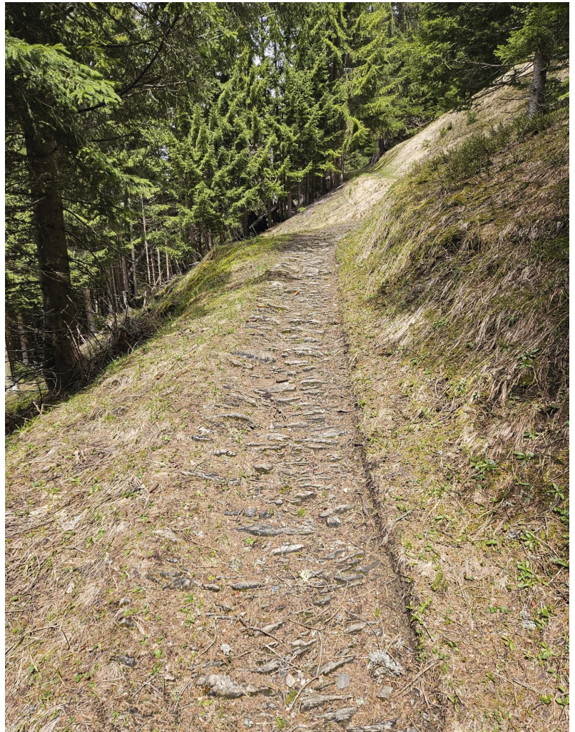
Fig. 3: Path in Safiental, between Stägä and Glasspass, built from local limestone set vertically into the ground (2024).
