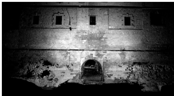
Figure 5: Point-cloud 3D model of (laser scanned) Nicosia's Venetian fortification (here, The Paphos Gate, situated on the infamous Green Line that divides the city since 1974).
