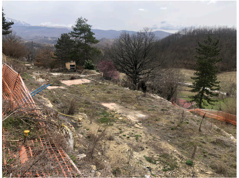
Fig. 4: The village of Poggio Vitellino after the 2016 earthquake destruction (photo 2022).
