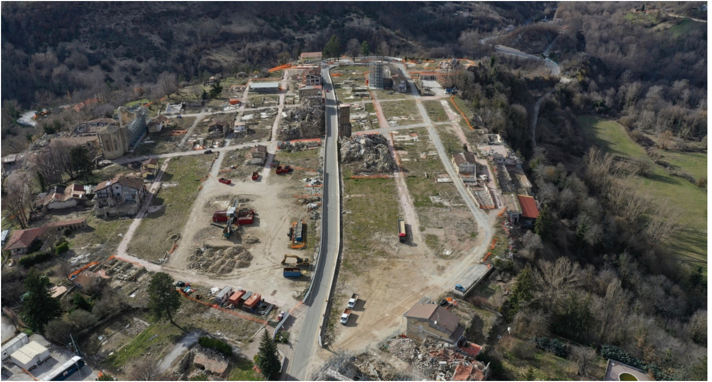
Fig. 1: City of Amatrice after the 2016 earthquake destruction (photo 2022).
