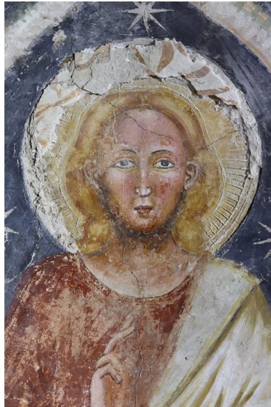
Fig. 1: Presentation of Christ in glory, mid-14th-century wall painting in the Chapel of St. Stephen, damaged by earthquake on 22 March 2022
