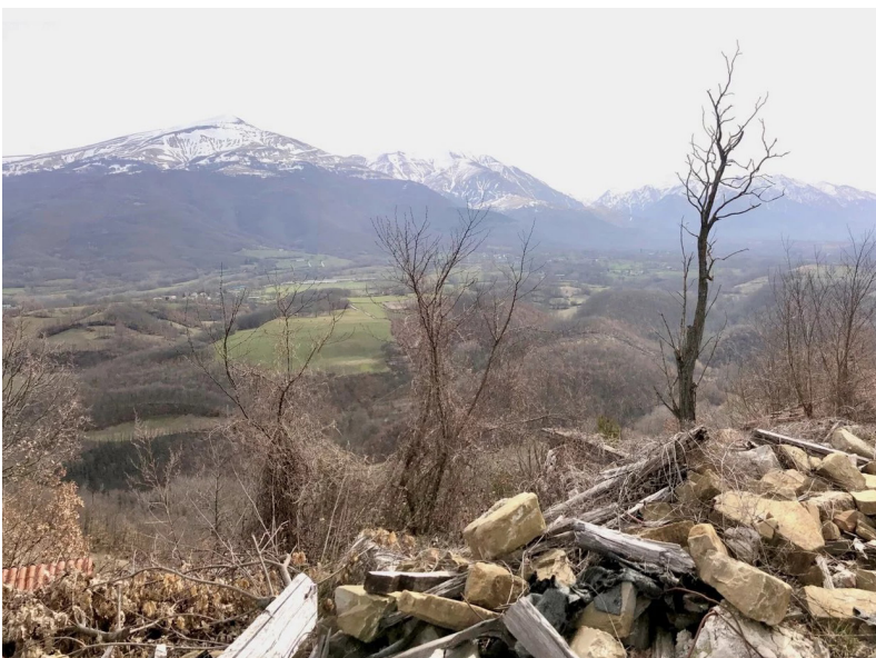
Fig. 3: The remains of the Poggio Vitellino’s church (photo 2022).
