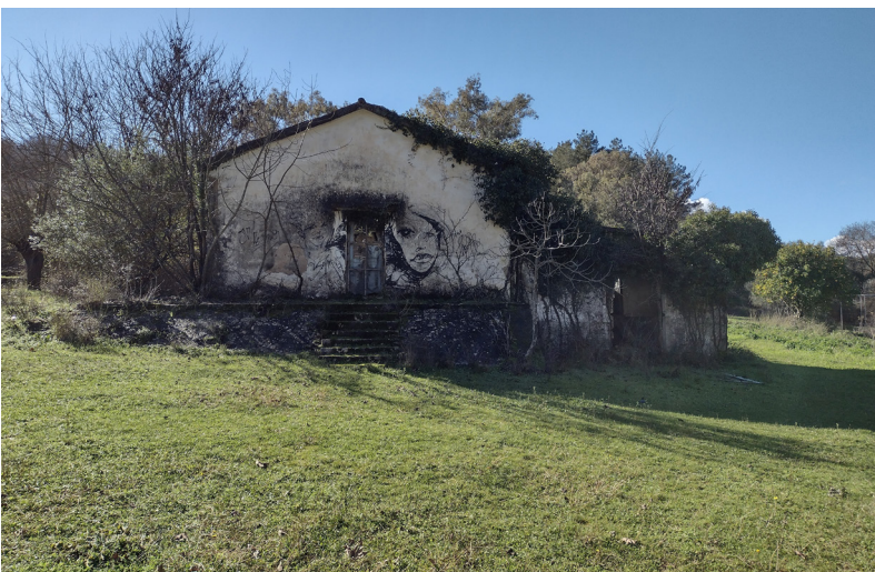
Fig. 4: Building in decay, Ziros Children's Town, Greece
