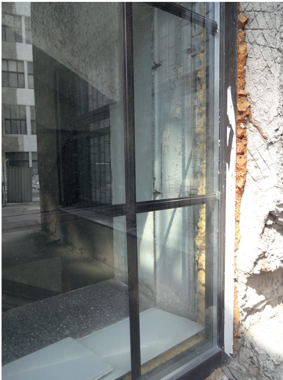
Abb. 14 Derzhprom: new replacement window frames, state 2014. Photo Svitlana Smolenska.
