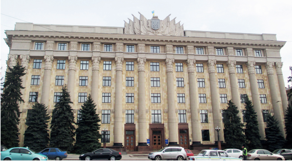
Fig. 9 The building of the Regional Committee of the Communist Party of Ukraine, 1955–1957, design by architects Veniamin Kostenko, Vladimir Orekhov, B. Miroshnichenko, Larisa Savenko; currently building of the Regional Administration, state 2013. Photo Svitlana Smolenska.
