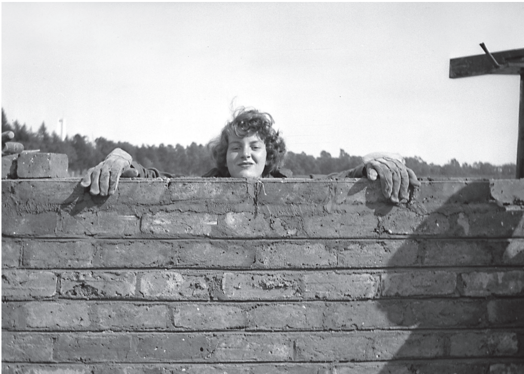
1 Denise Scott Brown, bricklayer on a student building project, Wits University, 1949, photograph by Clive Hicks
